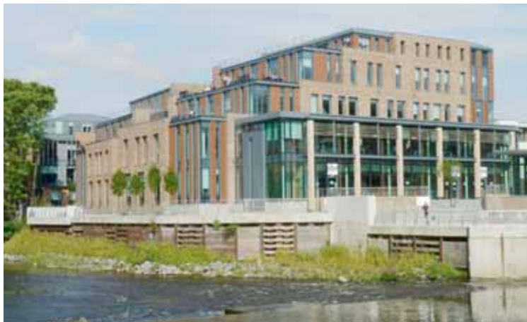
Freeman's Reach Office Blocks
