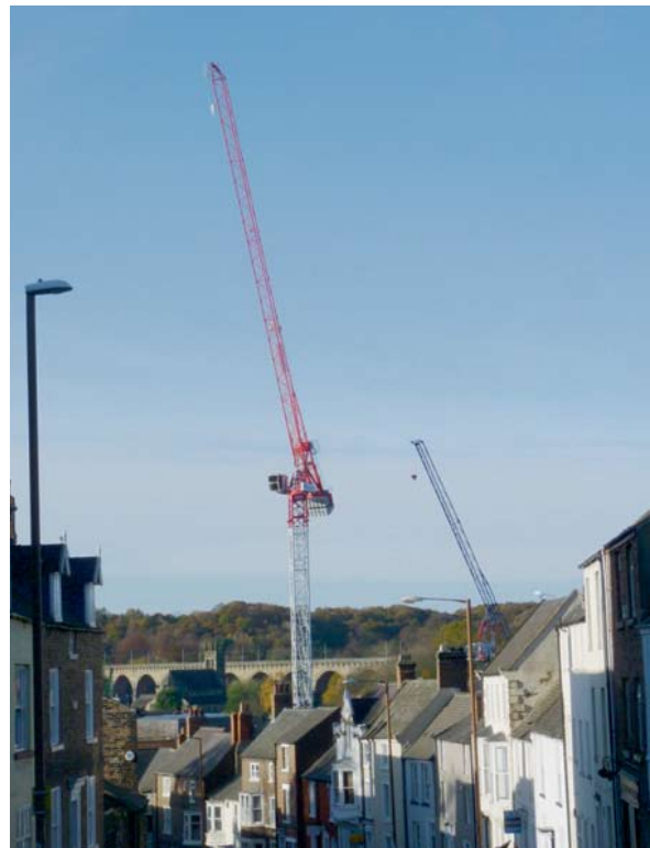
Jib-cranes in Lower Claypath
