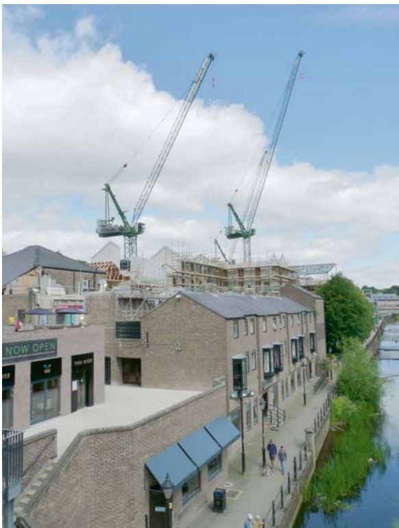
Jib-cranes over The Gates
