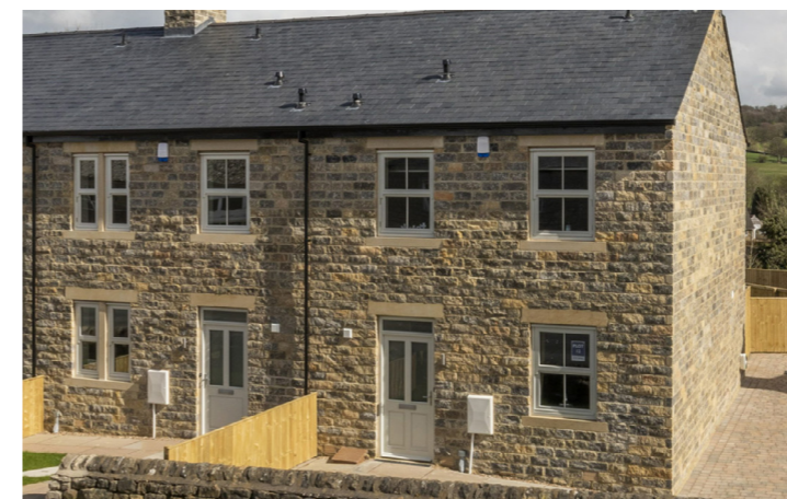
development reflecting local built form - Yorkshire Dales
