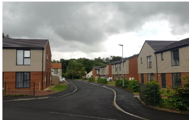
consistent material palette and detailing
