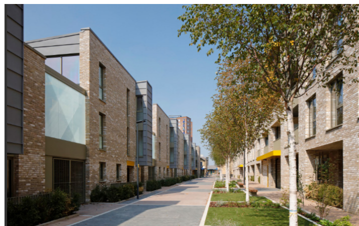
undercroft parking and landscaping ensures cars do not dominate the street - Priory Road, London (Housing Design Awards)
