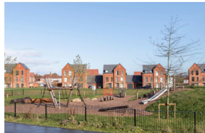
housing providing surveillance of open space and play area - Filwood Park, Bristol (Housing Design Awards)
