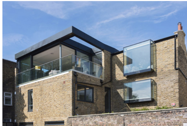
contemporary extension and box window (ODC Glass)
