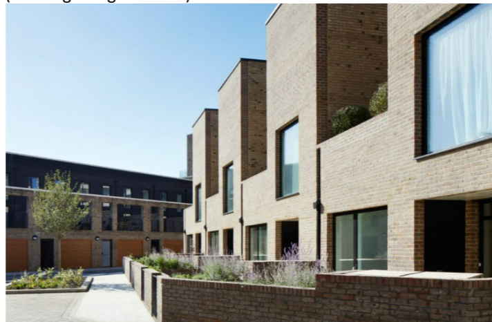
low brick boundary walls define private space (Housing Design Awards)
