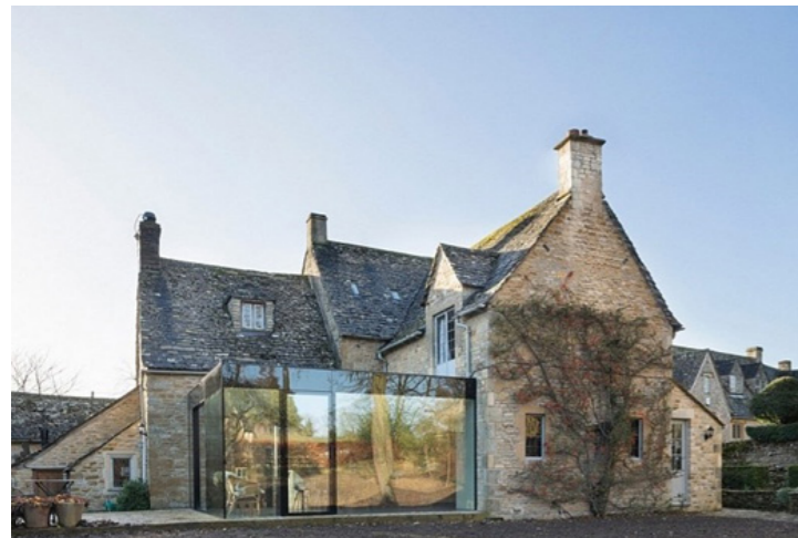
lightweight extension (Eastbrook Architects)
