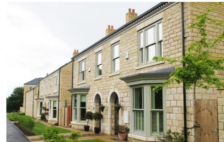
reference to local Georgian detailing and material palette (JRP)
