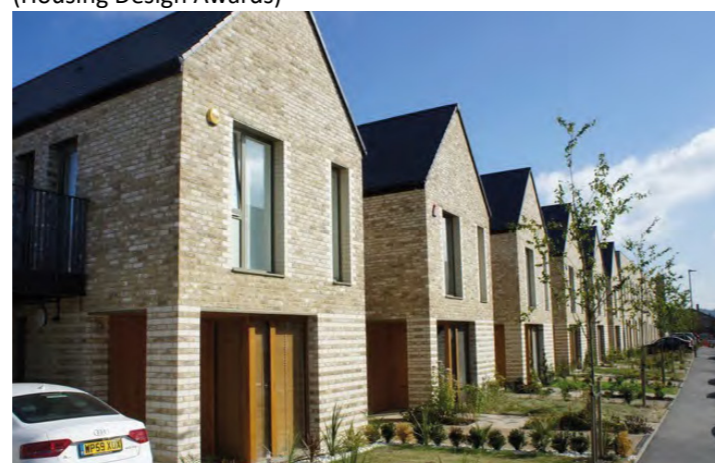
open garden, parking to the side (Building for a Healthy Life)
