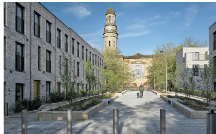
historic streets re-introduced to create permeable, well-sized urban blocks - Timekeepers Square, Salford (Housing Design Awards)
