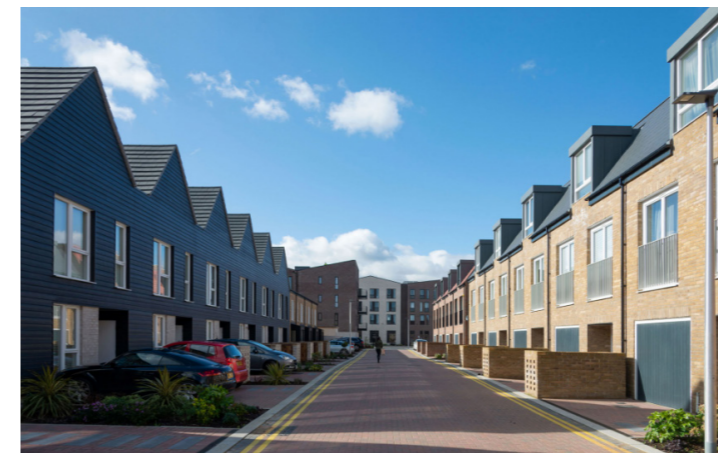
private space defined and parking screened by landscaping and boundary walls - Rochester (Housing Design Awards)
