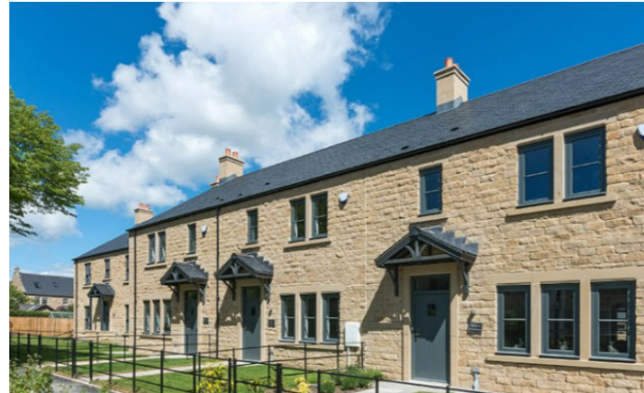
material palette and detailing responding to the historic estate - Belsay (County Life Homes)
