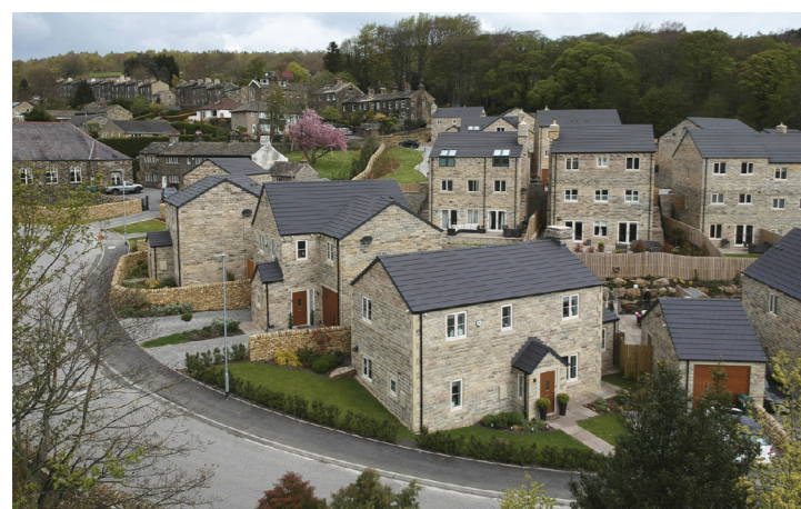
reference to local materials and boundary treatments - Bingley (LABC)
