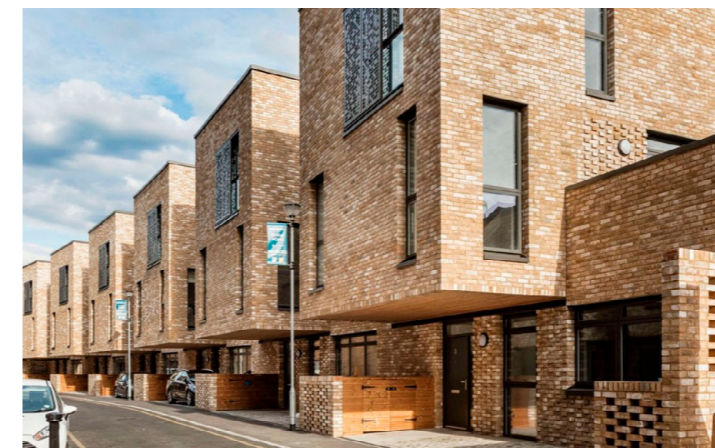
undercroft parking at back of pavement - Greenwich, London (BTPW)
