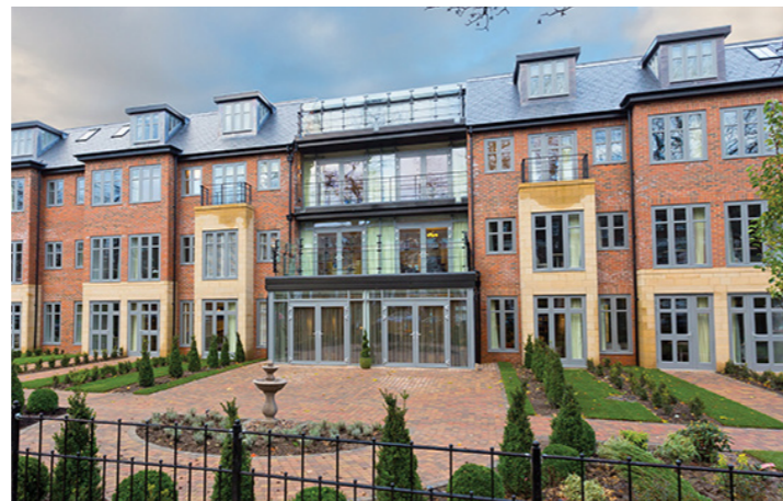
building form and scale responding to terraced street opposite (Helen McArdle)
