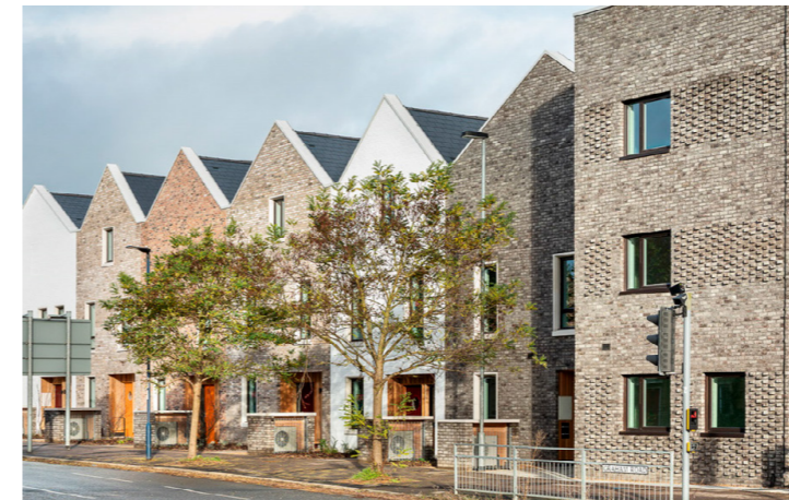
repetition of building form (Mole Architects)
