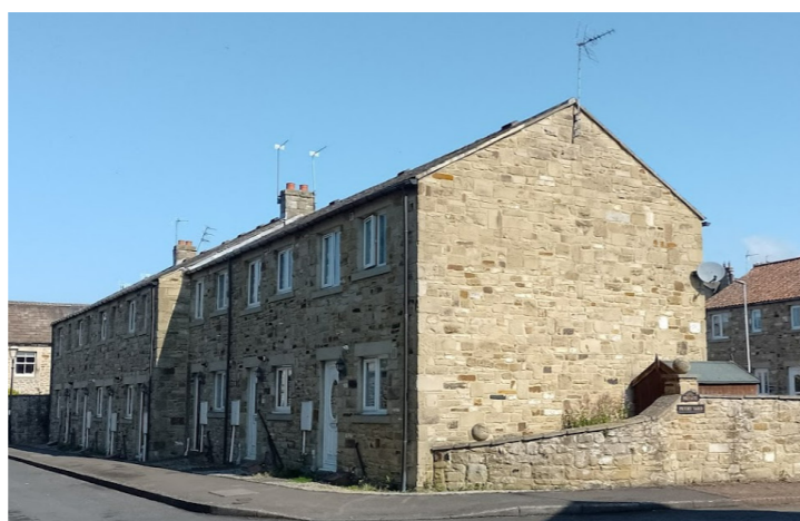
no boundary treatment to the front
