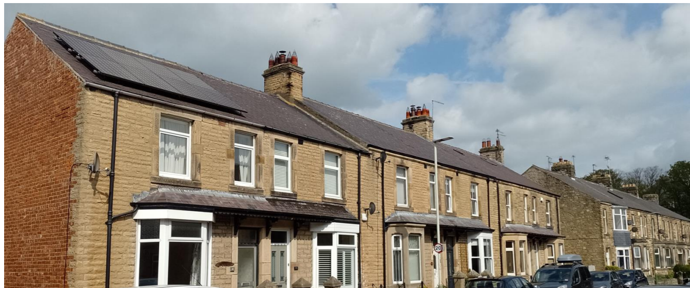
Solar panels on terraced street
