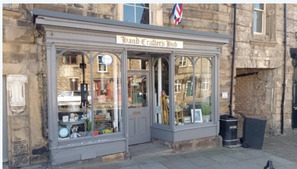
Timber shopfront with stone base to stallriser
