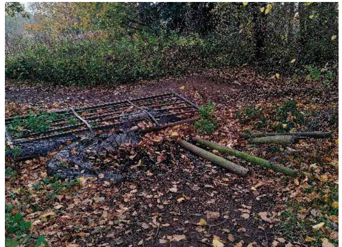
Tumbledown metal gate and fencing at copse
